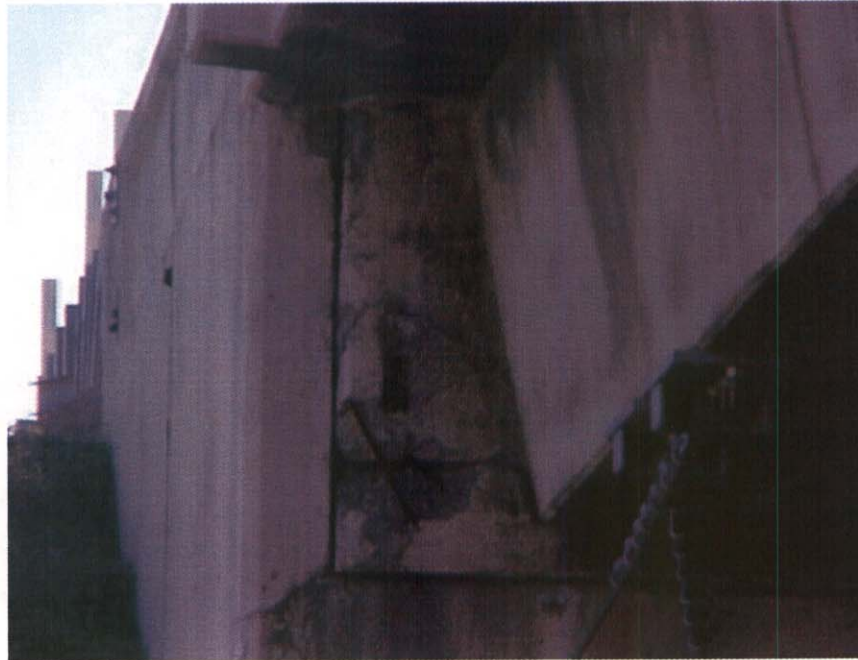
ABUTMENT #2 BACKWALL SPALLED
