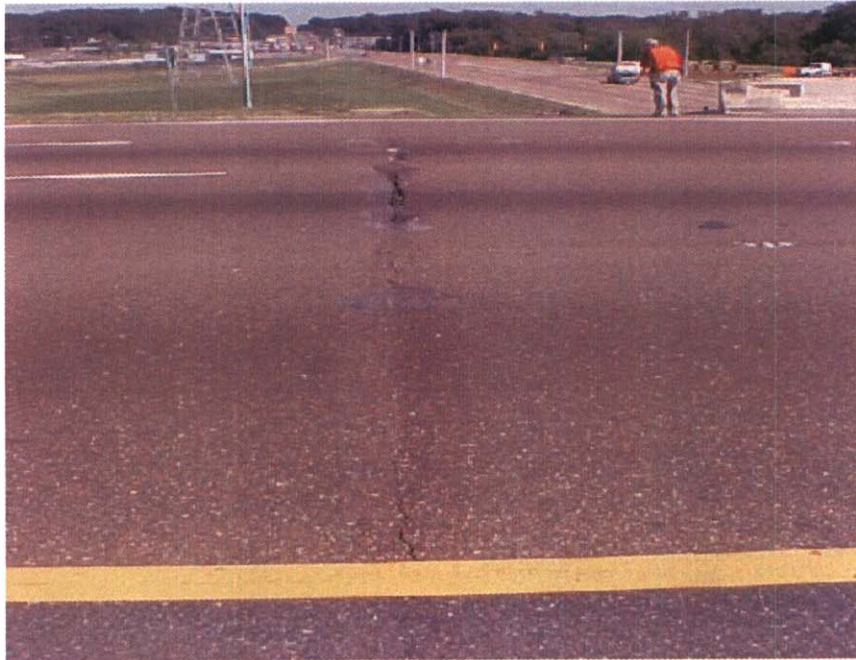
APPROACH #1 JOINT SPALLED
