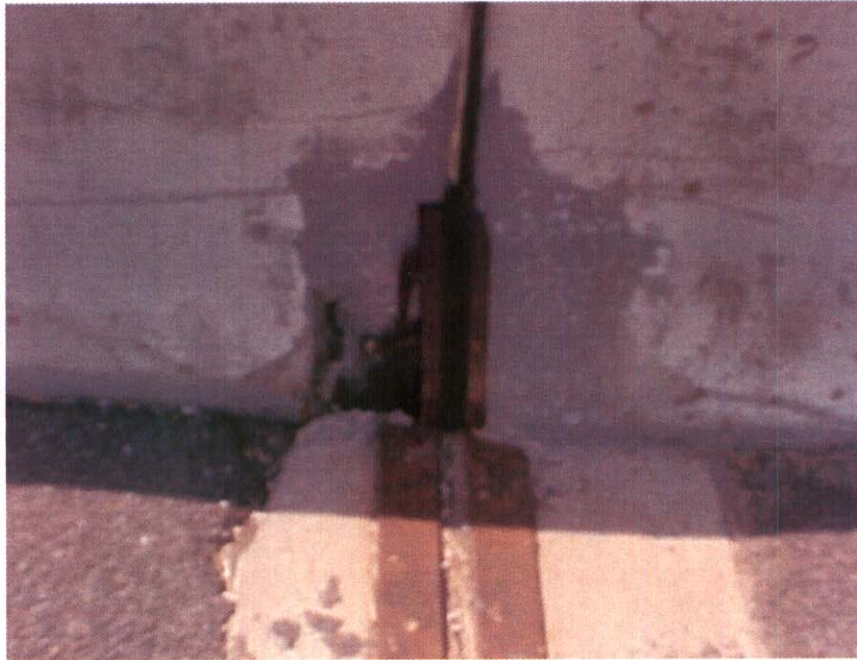
APPROACH #2 PARAPET SPALLING AT JOINT
