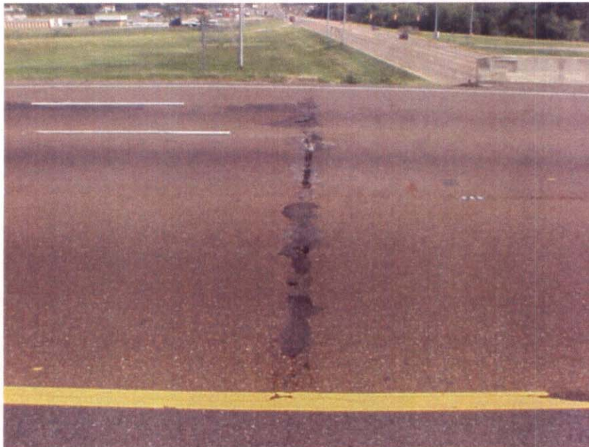
APPROACH #2 WITH ASPHALT SPALLING
