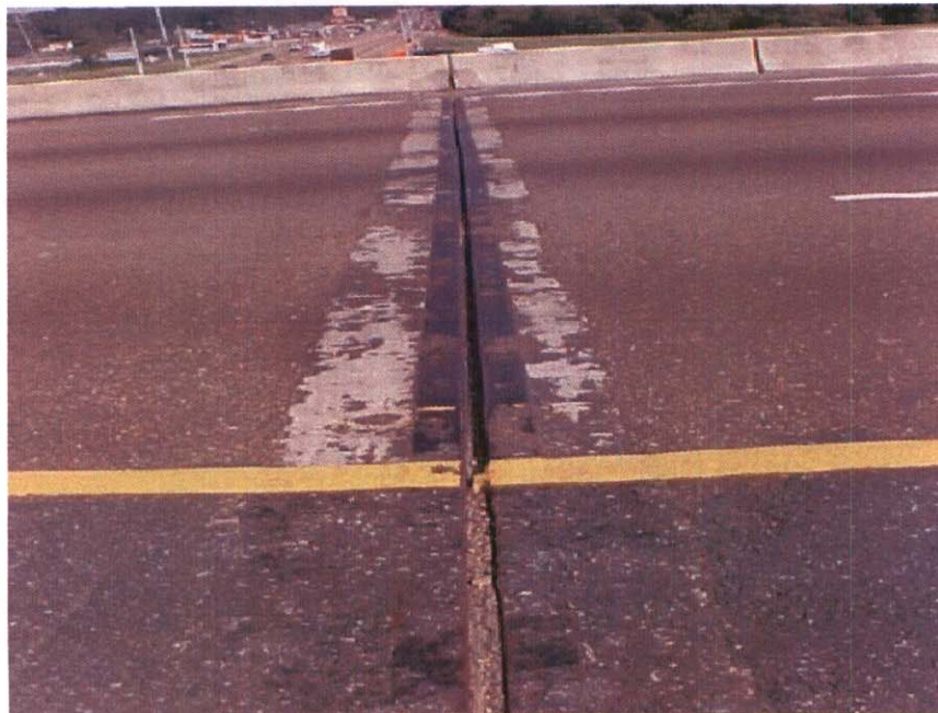
APPROACH #2 PARAPET SPALLING AT JOINT
