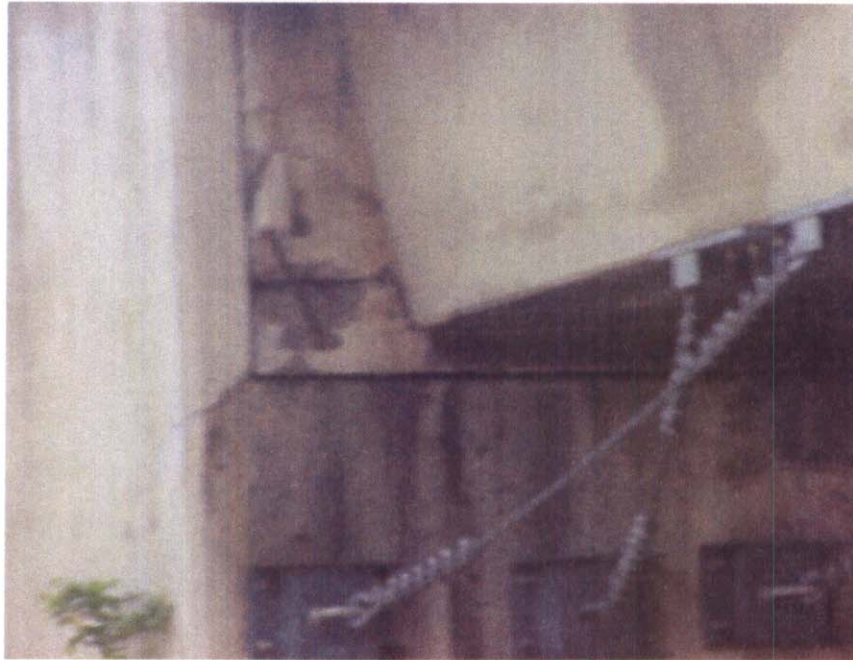
ABUTMENT #2, LEFT BACKWALL SPALLED TO STEEL
