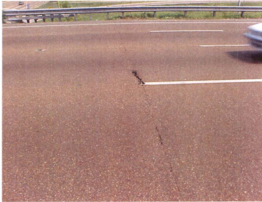
APPROACH #2 WITH ASPHALT SPALLING
